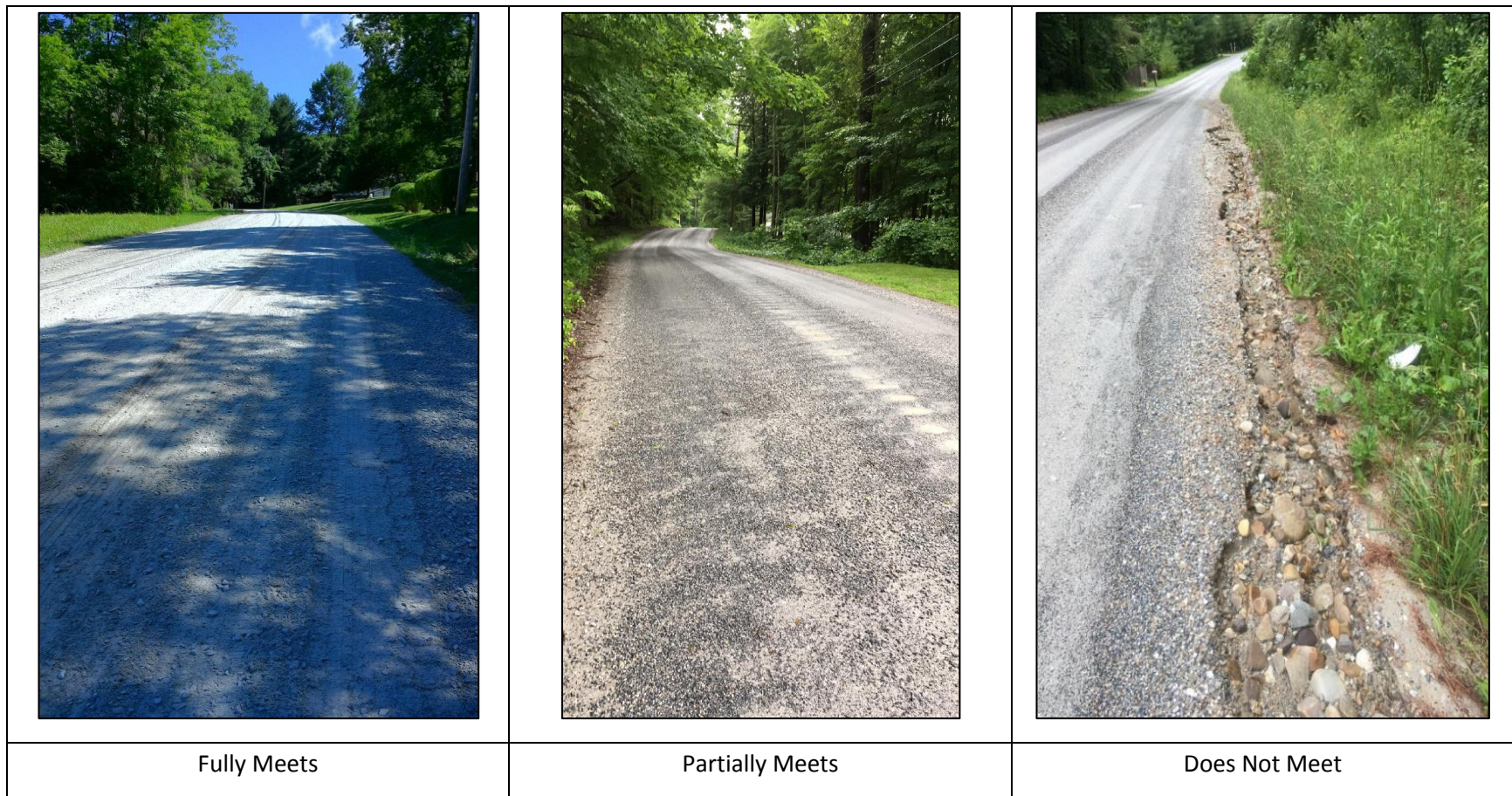
Figure 4.4: Examples of road segments with different levels of MRGP compliance.
