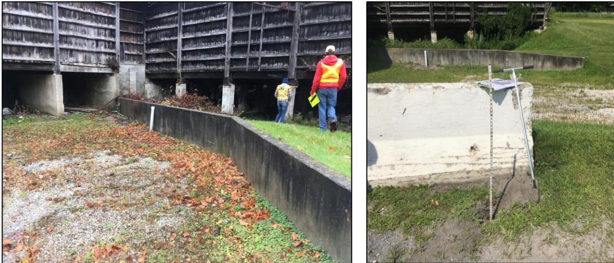
Figure 5.3: Exploring drainage patterns and discovering a buried catch basin during concept design development in the Chittenden Drive area (SW-7 & SW-8).
